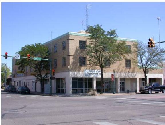
14. 201-203-205 S. Main St. 5PW.352 Maxwell House Hotel 1938
